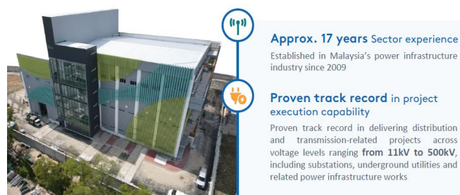
Figure 22: SKA at a Glance: 17 Years of Track Record from 11kV to 500kV
