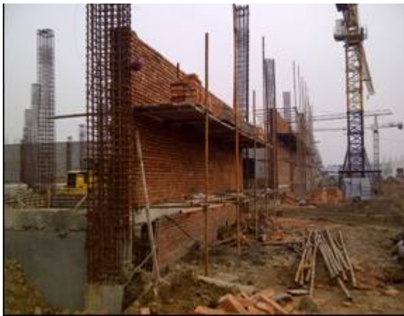
“Construction site for Sozo’s new 3rd factory”
