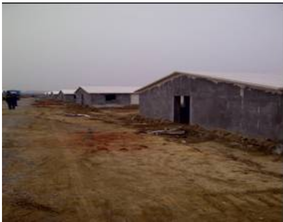
“Under construction – exterior of duck housing”
