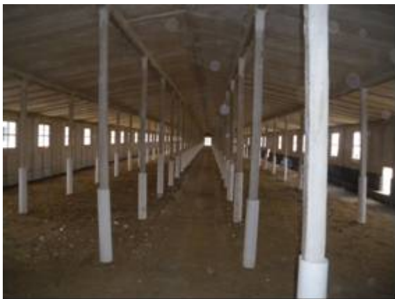
“Under construction – interior of duck housing”
